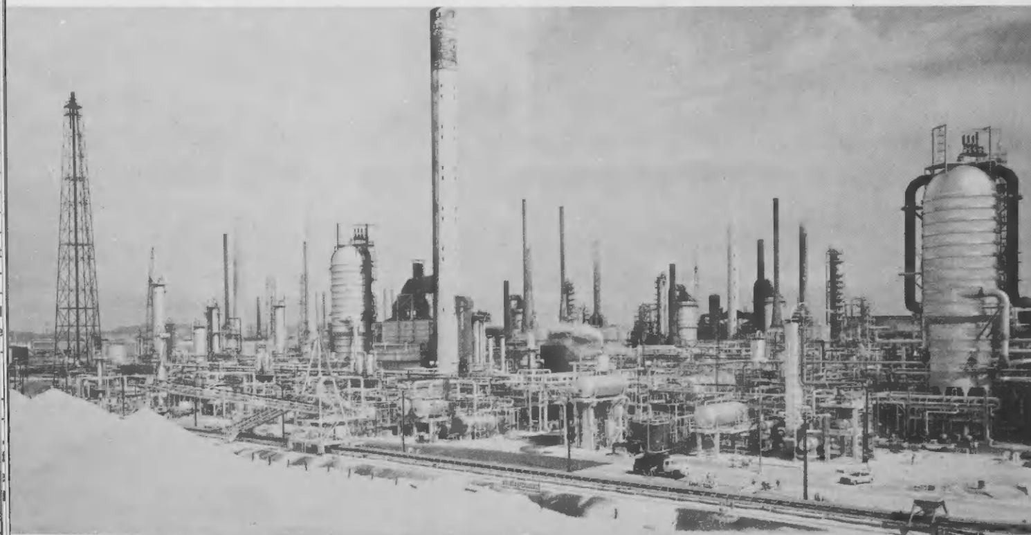
Lago's HDS Facilities.
